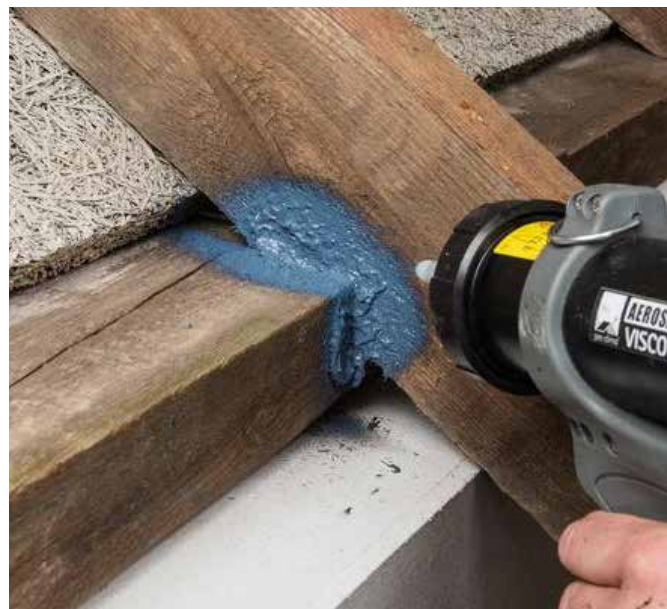
Simple airtight sealing of penetrations e.g. collar ties or rafters when carrying out roof refurbishment from the outside.
