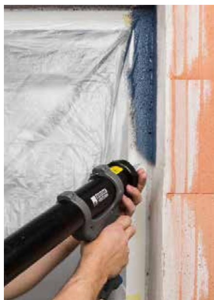
Creation of airtight interior airtight joints and exterior joints that are resistant to driving rain, using either a painting or spraying procedure. Can be used flexibly on fibrous insulation materials (e.g. hemp wool or sheep wool) and on spray foam. Interior and exterior joints tested and confirmed in accordance with the IFT Guideline MO-01/1:2007-01, Section 5.
