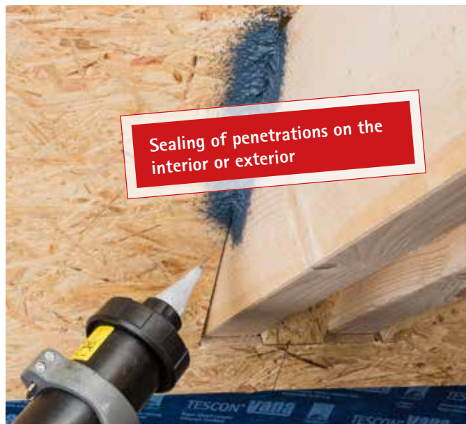
Simple airtight sealing of penetrations e.g. collar ties or rafters when carrying out roof refurbishment from the outside.
