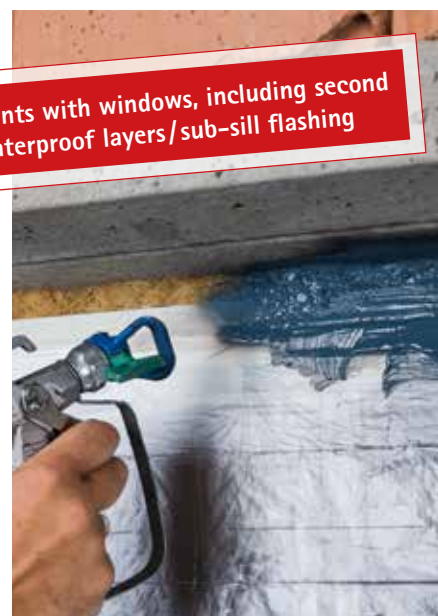
Creation of airtight interior airtight joints and exterior joints that are resistant to driving rain, using either a painting or spraying procedure. Can be used flexibly on fibrous insulation materials (e.g. hemp wool or sheep wool) and on spray foam. Interior and exterior joints tested and confirmed in accordance with the IFT Guideline MO-01/1:2007-01, Section 5.
